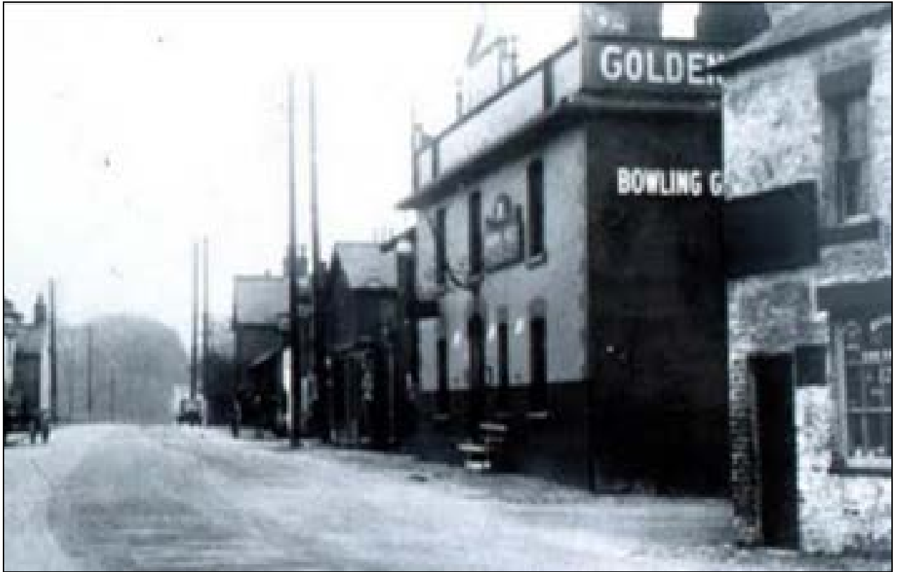
The building subsequently underwent alteration, with addition of a parapet and render
